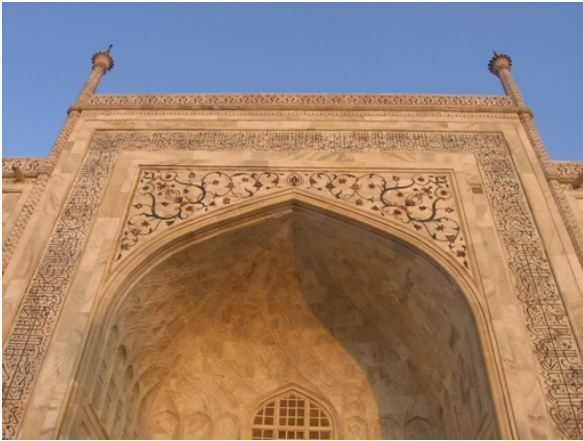
Detail of the west elevation showing inlay of semi-precious stones and Islamic calligraphy of texts from the Koran
